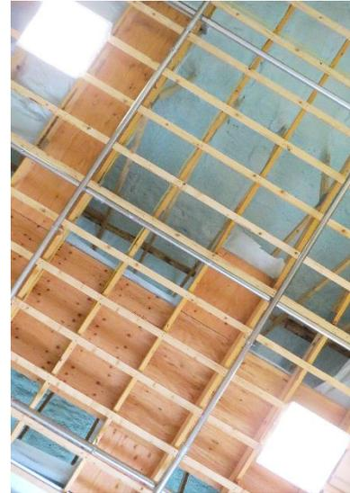
Suddenly, all that changed. This week we installed the foam soundproofing. It’s sprayed onto the ceiling and walls to a depth of about six inches, providing excellent thermal insulation and sound deadening. The room looks and sounds different now. It’s not a nondescript empty space anymore. It’s a TV studio. The echo of hollow emptiness is gone. As large as it is, the foam’s acoustic diffusion makes it more intimate, quieter.
