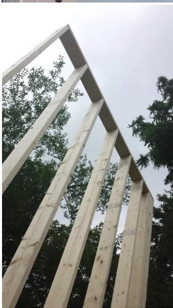
The walls rise to 16 feet. In our 32' x 32' studio the height is necessary to have ample room to mount studio lighting above the larger sets that this room can accommodate. I took this photo from the roof of our trailer.
