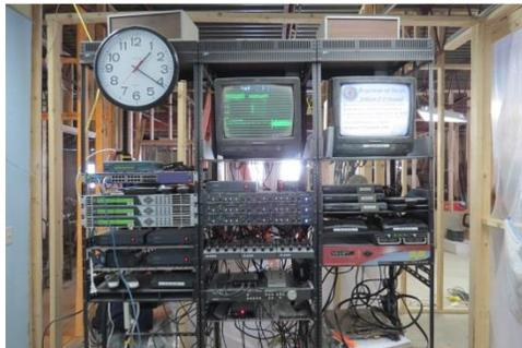
Next, we remove the temporary plastic frame and roll our racks - all still connected and working - to their new temporary position so Keith and Adam can finish framing the surrounding walls.
