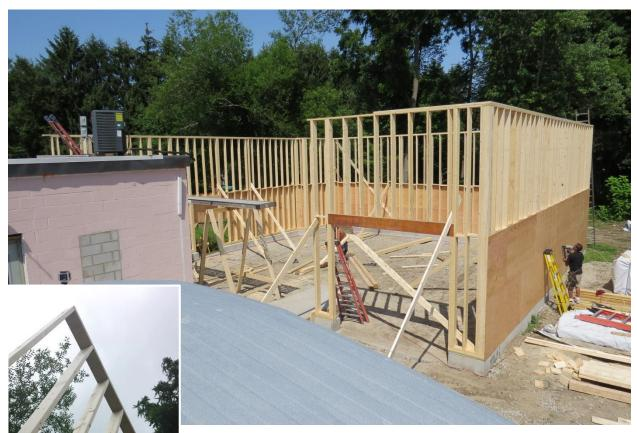
The walls rise to 16 feet. In our 32'x 32' studio the height is necessary to have ample room to mount studio lighting above the larger sets that this room can accommodate. I took this photo from the roof of our trailer.
