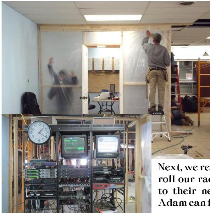
Next, we remove the temporary plastic frame and roll our racks - all still connected and working - to their new temporary position so Keith and Adam can finish framing the surrounding walls.
